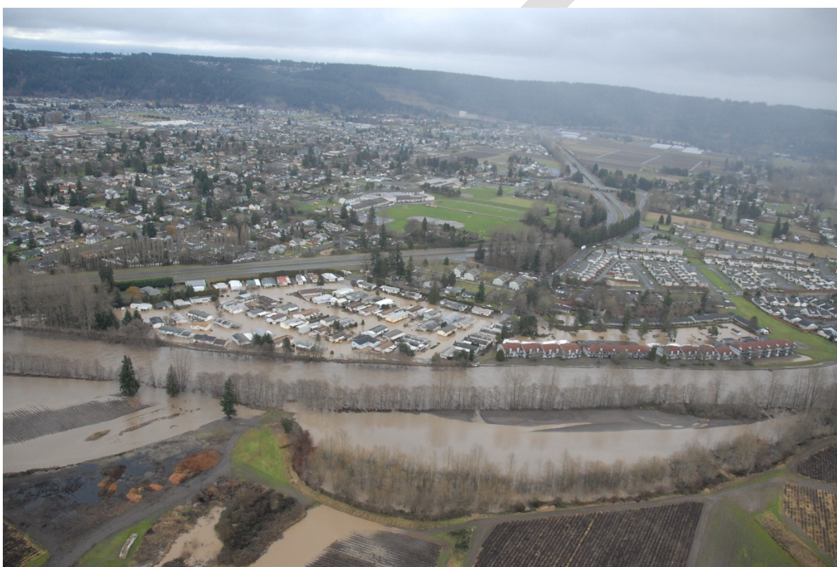
Figure 2-1. Looking northeast across the Puyallup River near RM 11.2 (January 8, 2009)
